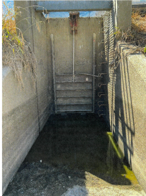
Figure 2: Duck Creek Headworks
