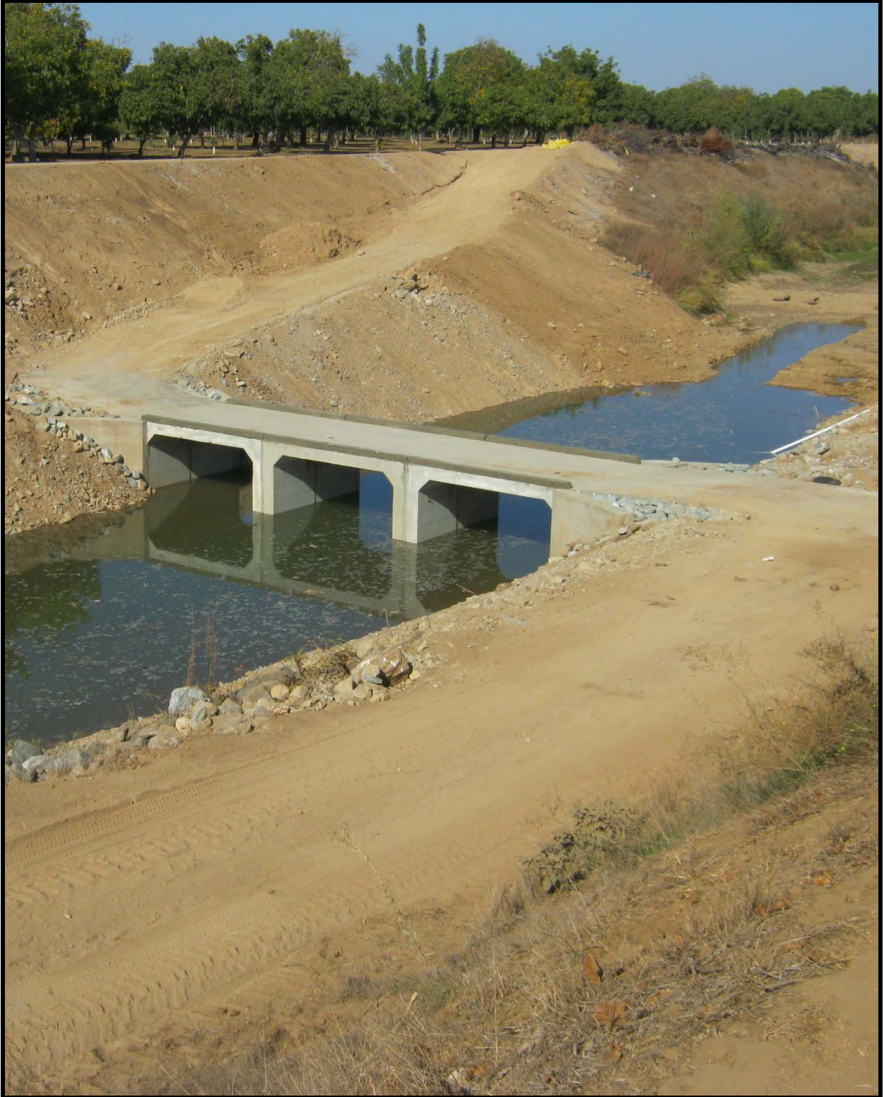
FIGURE 3 Low Water Culvert Crossing Example
