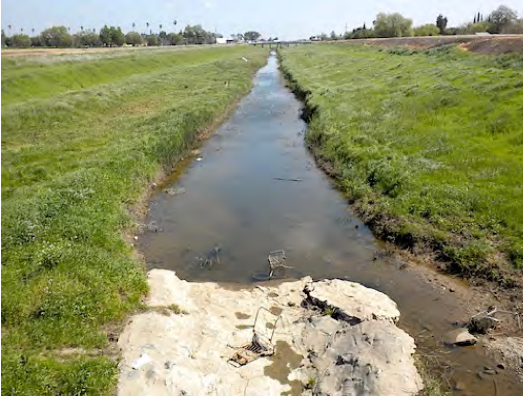
Photo 5. Looking upstream from the Central California Railroad Crossing.
