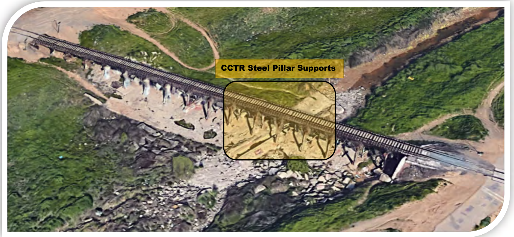
TRAIN TRESTLE SITE MAP AND CONSTRUCTION NEAR STEEL PILLAR SUPPORTS
