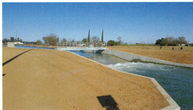
Figure 2: Replogle Flume
