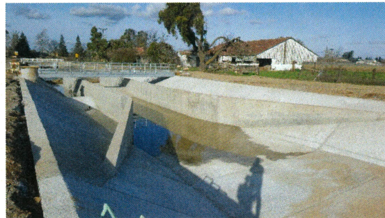
Figure 1: Empty Replogle Flume
