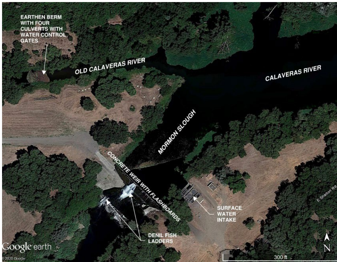
Figure 4.10-1. Prominent Features of the Bellota Weir Modifications Project Site
