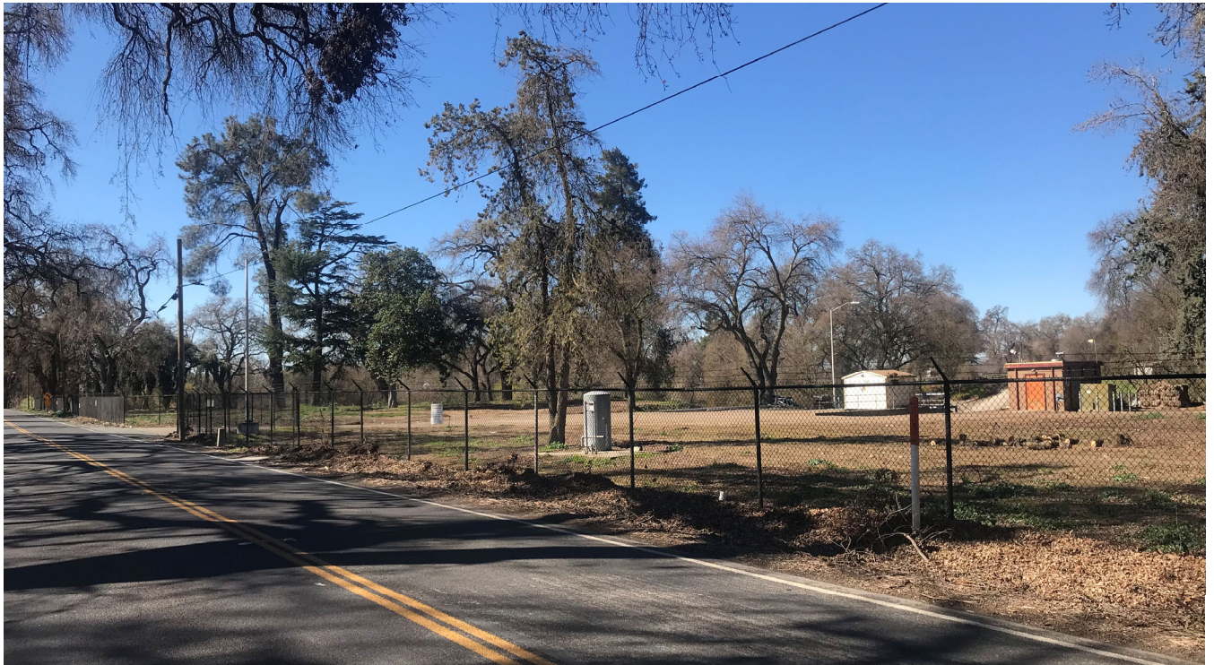
Photo Plate H: Existing view of Project site from East Shelton Road looking southwest. Existing East Entrance is shown on photo left. Existing Project site structures are shown on photo right. The existing Bellota Intake is out of view located just beyond the existing structures below the Mormon Slough top of bank.
