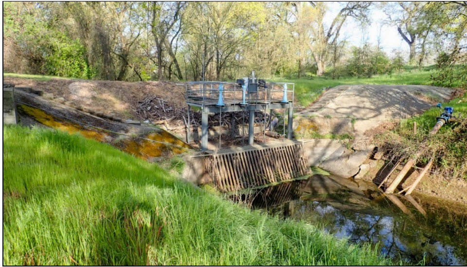
Figure 4.4-7. The current configuration of the Old Calaveras Headworks at low flows.
