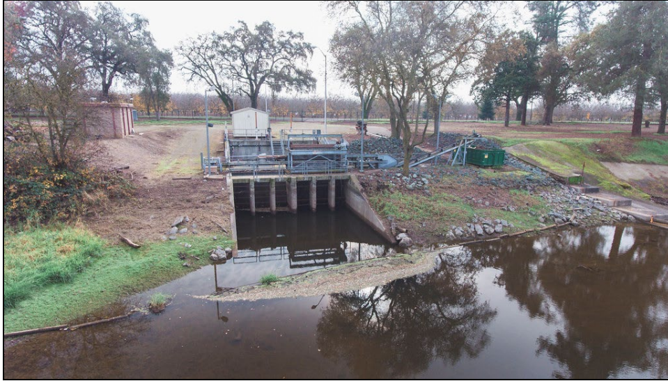
Figure 4.4-1. Current configuration of the Bellota Intake.
