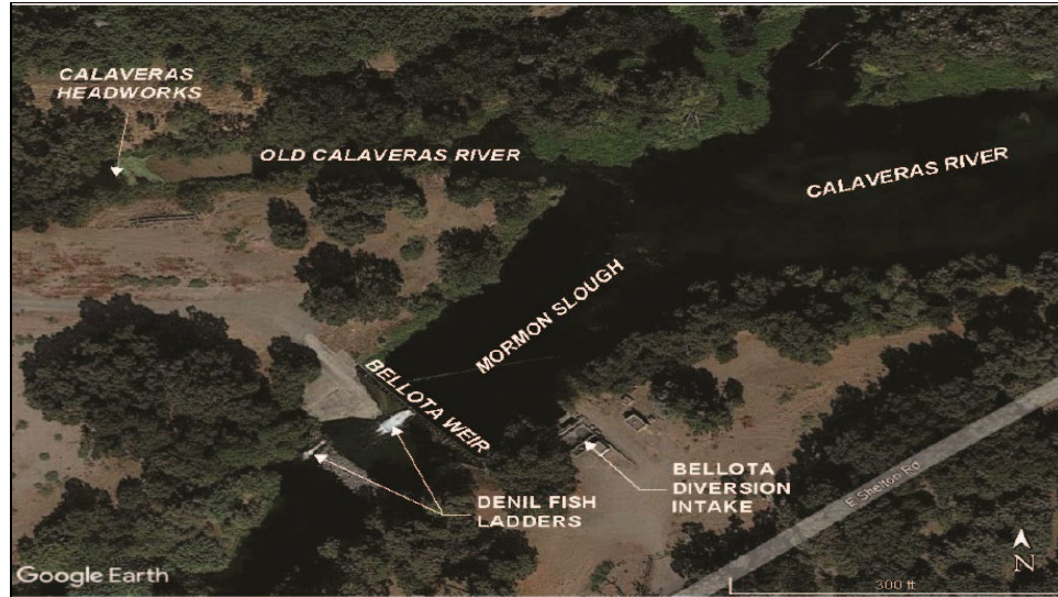
Figure 4.4-5. Aerial view of the current configuration of the Project Area.
