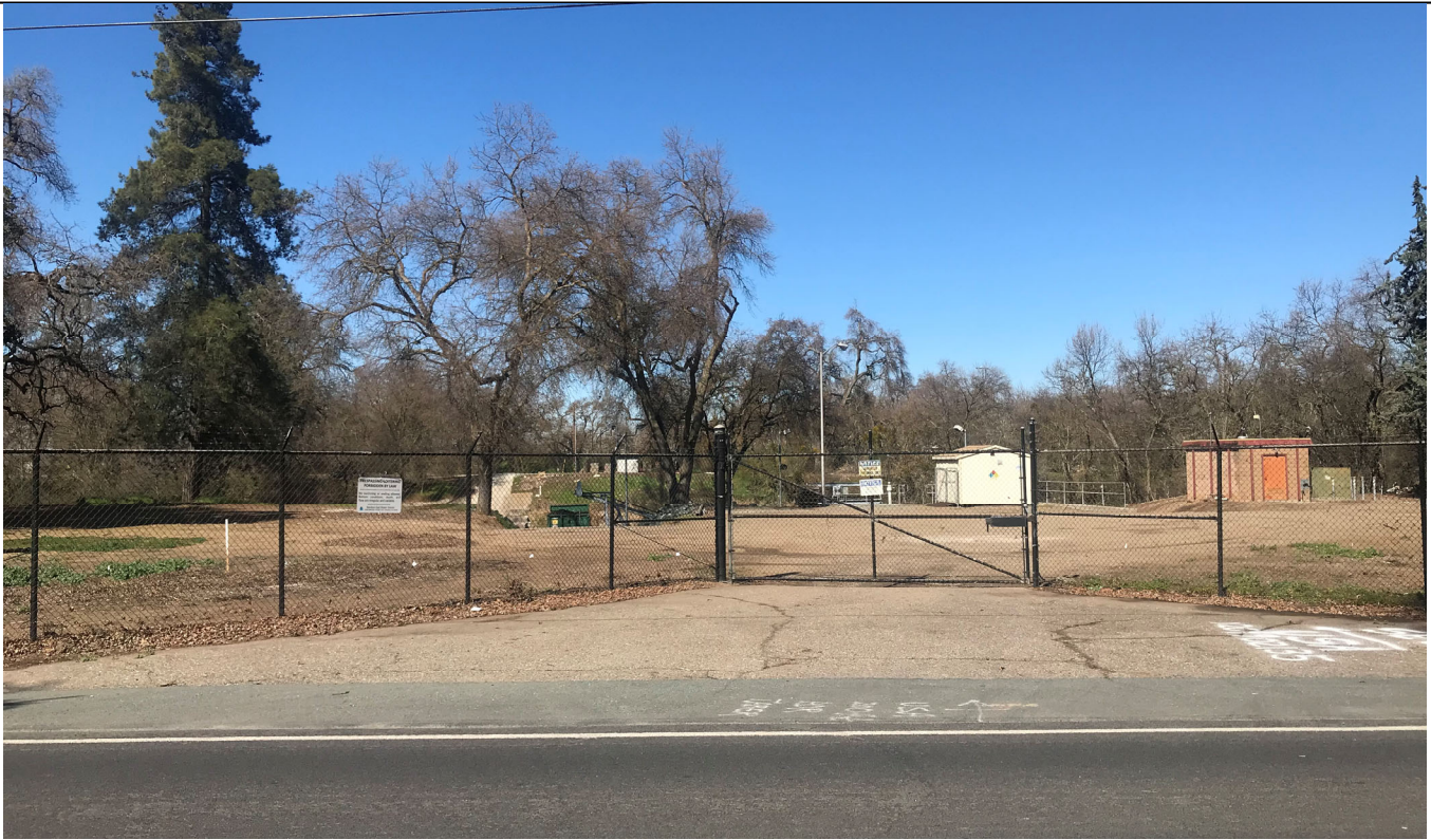
Photo Plate G : Existing view of Project site East Shelton Road entrance looking northwest. Existing Bellota Intake and trash racks are out of view located just beyond the small structures below top of bank. The existing Bellota Dam concrete apron located on Mormon Slough north bank can be seen in the background.
