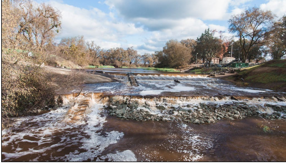
Figure 4.4-2. Photo of Bellota Weir from ground level during high-flow event.
