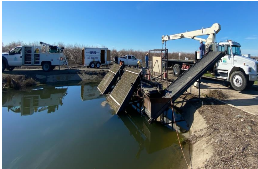
Figure 1. IWS is replacing the screen chain drives with direct drive gearboxes
