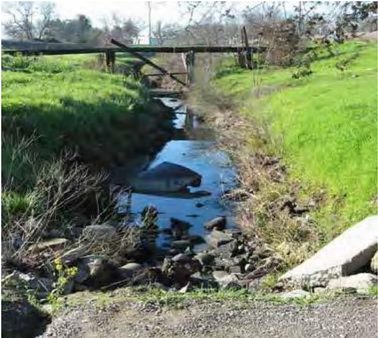
Figure 1. Old Calaveras downstream of Gotelli Low-flow Road Crossing. Photo from DWR 2007.
