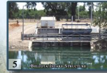
5 Belleta Intake Structure
