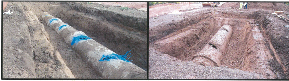
Photos 1 and 2 showing damage to top of 54-inch RCP Bellota Pipeline.
